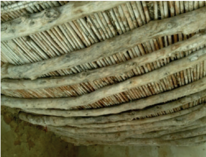
Figure 11: Logs and reeds in a Traras house roof.
